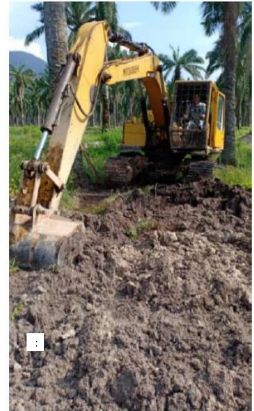
Figure 1 Excavator bucket tilting the soil
