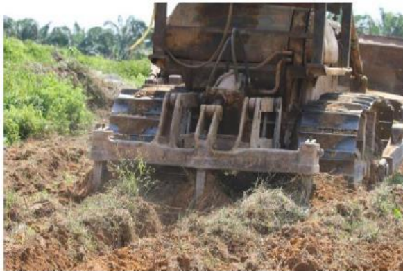
Fabricated steel ripper mounted on D6 bulldozer
