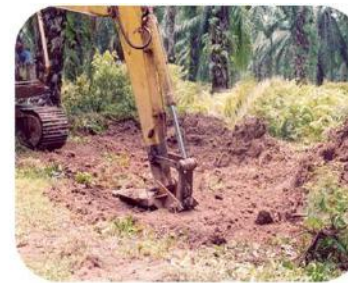
Step 4: Filling up the deboled area with nearby soil or new soil.
