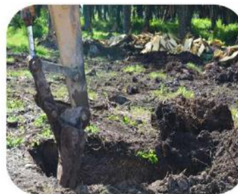
Step 3: Excavating stump and root mass at length of 1.5 m x 2.0 m, width of 1.5 m -2.0 x & depth of 1.0m -1.5m
