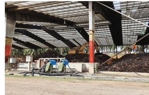
POME – EFB mixing process ( POME spraying and EFB turning using a backhoe)
