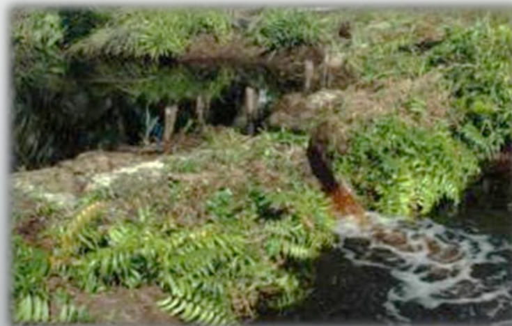
Adjustable weirs made from sand bags to increase water-table to 15-30 cm
