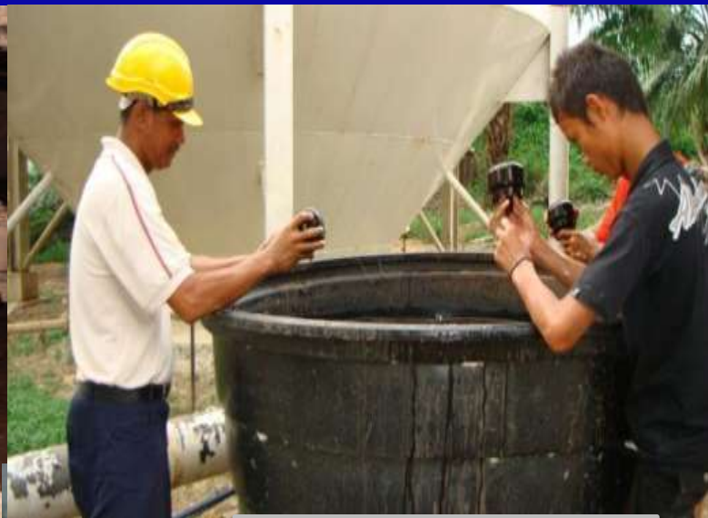
MANUALLY CLEANING THE DIFFUSER
