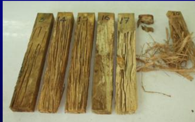
Excavation patterns of several termite species
